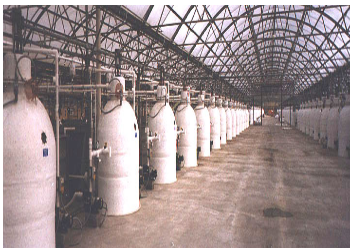
Bead Filters at a Large Midwestern Tilapia Facility (Malone et al)
